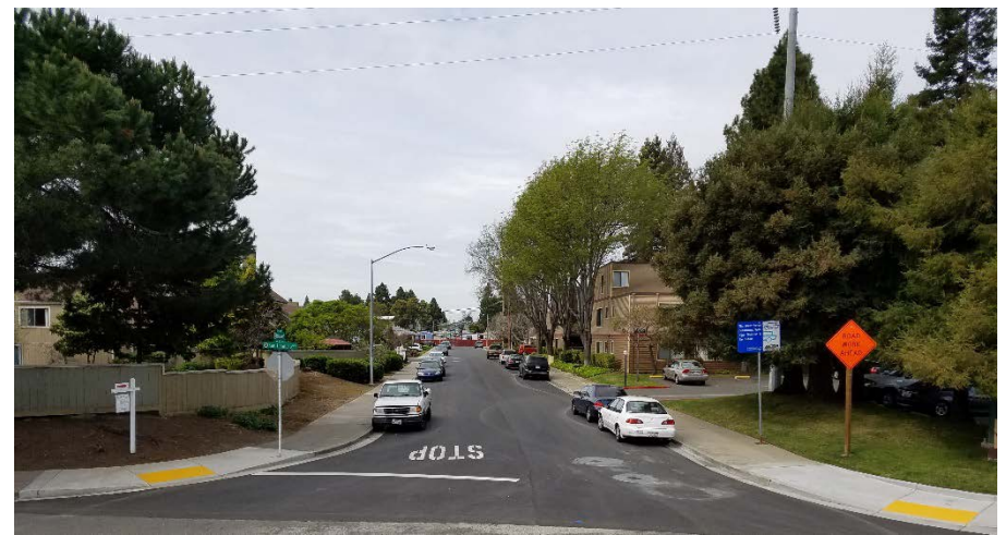
ROSE DRIVE (FULL DEPTH REHABILITATION)
